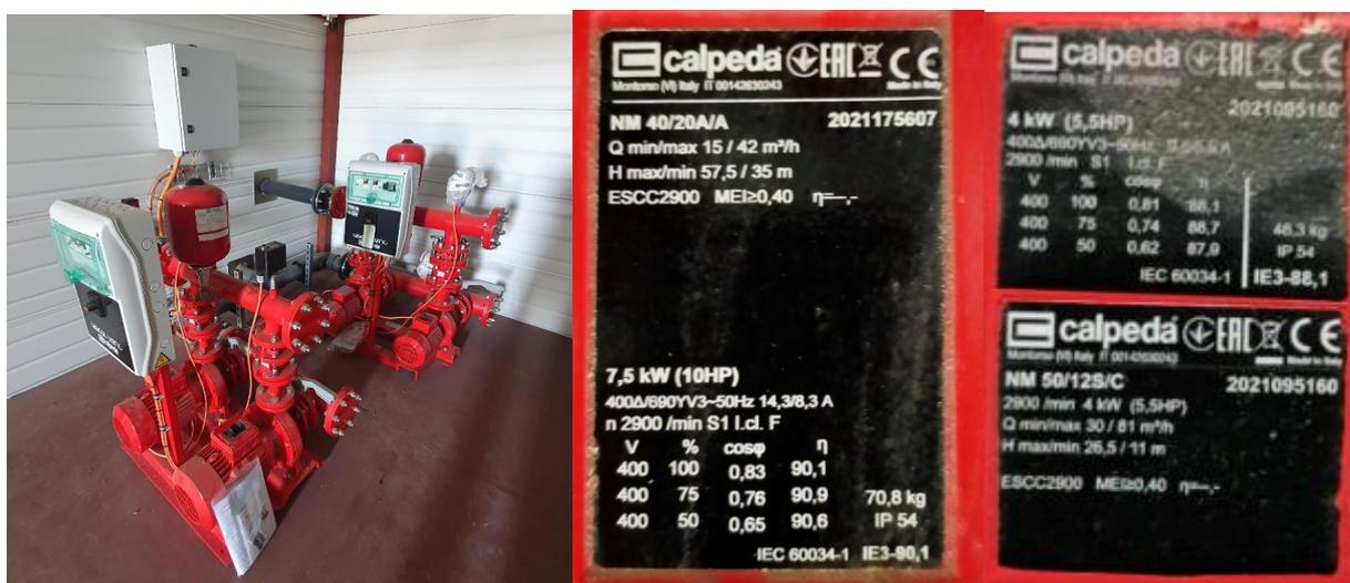
**PHOTO 15 : DOUBLE SYSTEME DE POMPES POUR ALIMENTER LE RESEAU D'INCENDIE**
