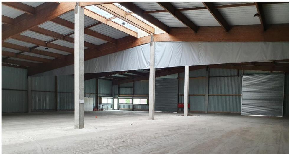
**PHOTO 11 : DISPOSITIF DE DESENFUMAGE INSTALLE DANS LE BATIMENT 2 ET ECRANS DE CANTONNEMENT EN COURS D'INSTALLATION**
